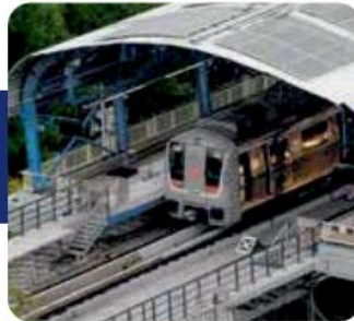
Delhi Metro Rail Corporation
