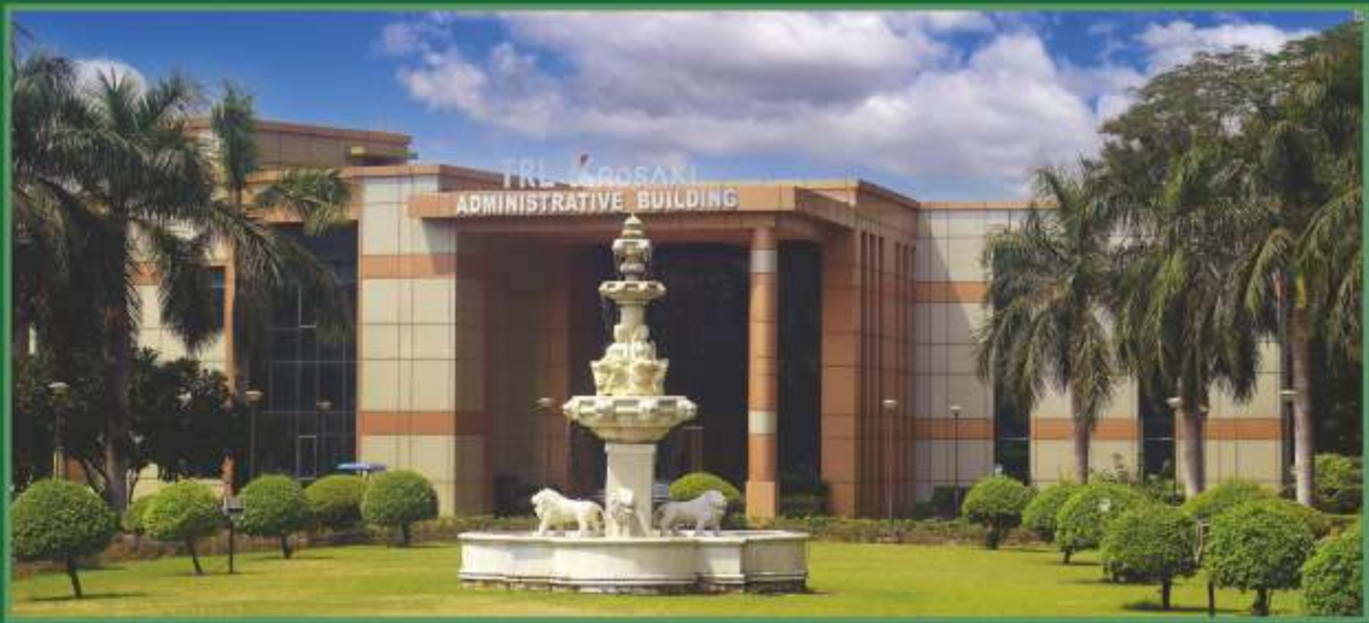
Administrative Building, Belpahar
