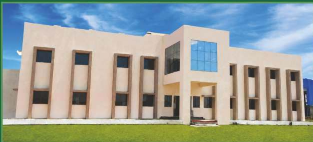
Administrative Building, Gujarat Works
