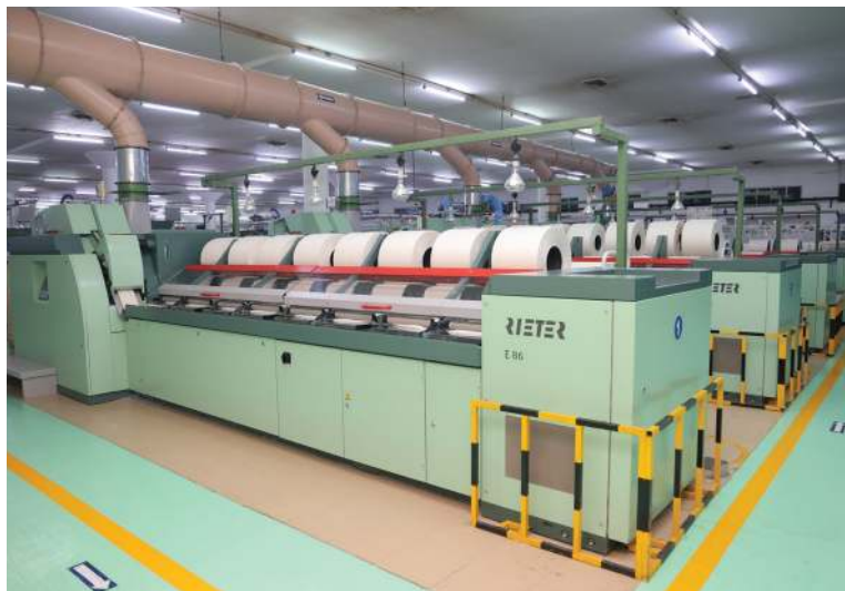
A view of new "Rieter E86" Comber Machine installed in our Unit at Rajapalayam.
